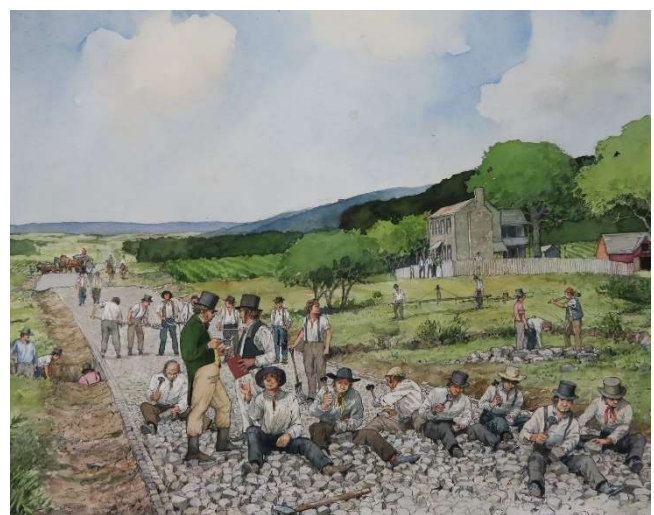
A painting of the macadam process commissioned by the Foundation, depicting the installation of the Boonsboro-Hagerstown Turnpike Road.
