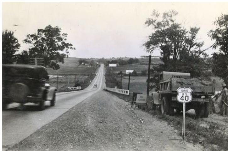
A stretch of Rt.40 nearing the end of improvement work.
